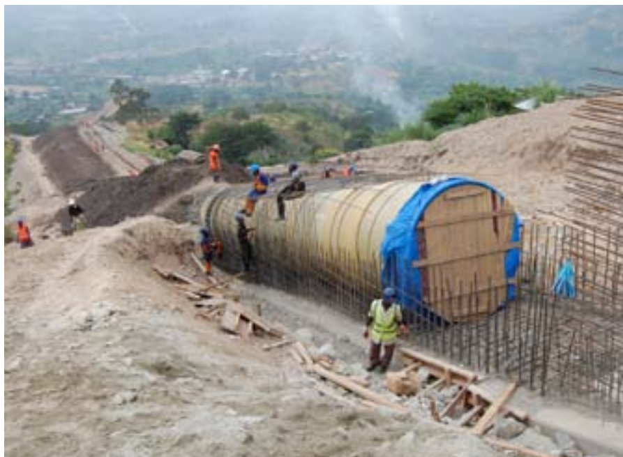
Construction work at hydropower plant Bugoye, Uganda.
